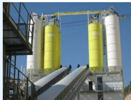
Pneumatic transport for cement and ash to different destinations. Continuous supply to plant.
